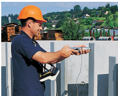
Series testing of prefabricated concrete elements with automatic data storage
